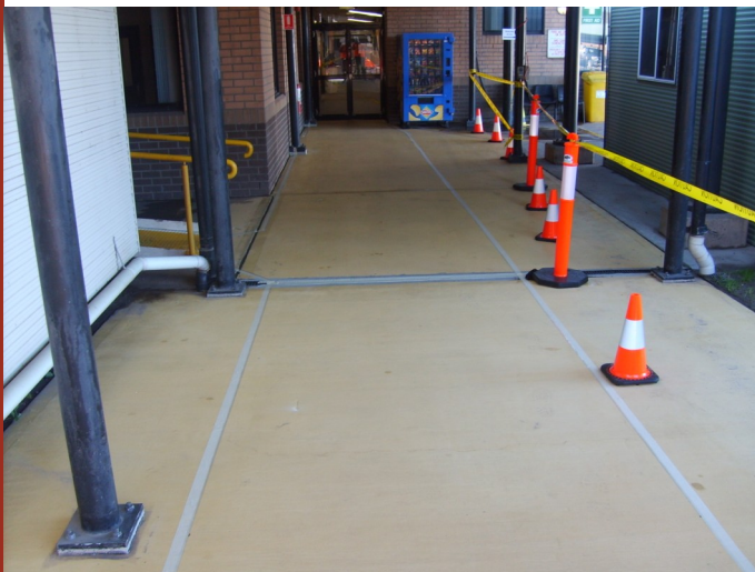
3. Dried and prepared for ArmaFloor application
